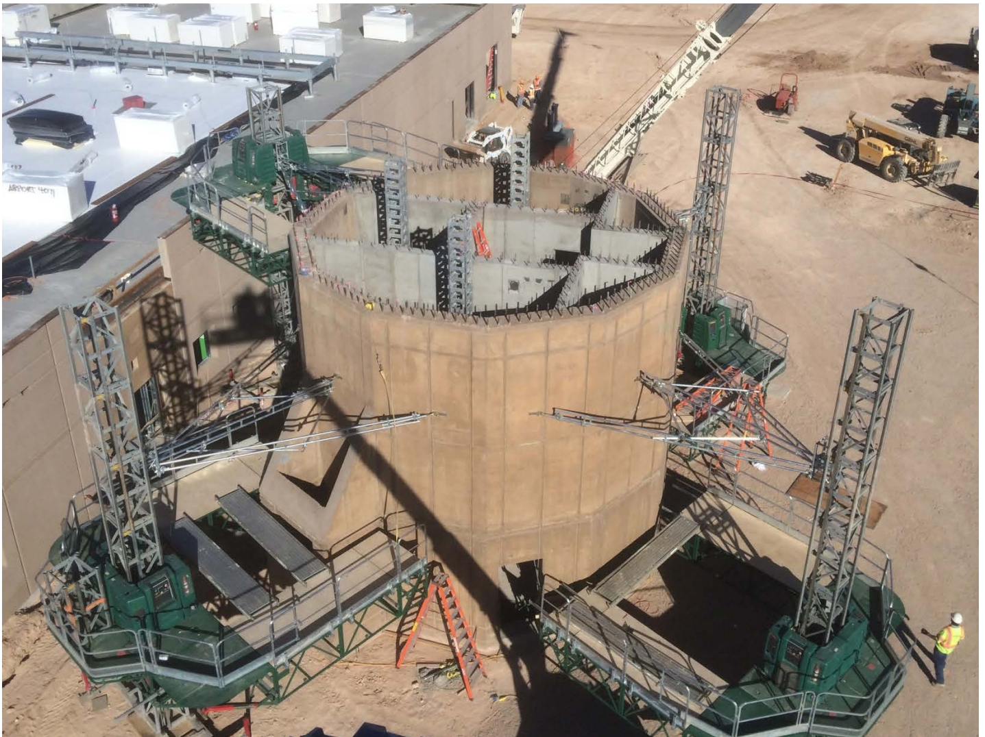
FULL CONSTRUCTION SET-UP SHOWING FOR EXTERNAL AND THREE INTERNAL UNITS
